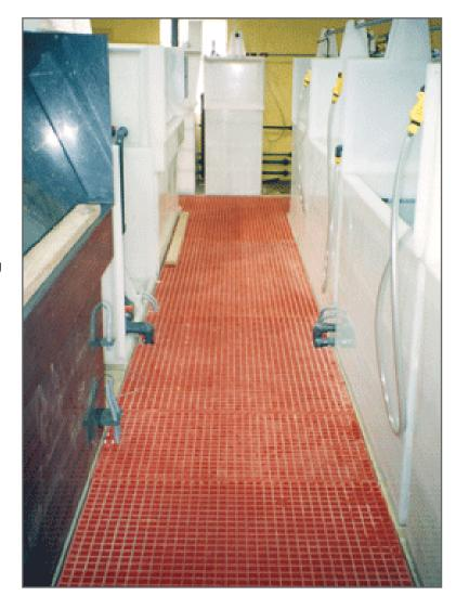
Fibergrate supplied 1" deep, 1-1/2" square mesh Vi-Corr® fiberglass reinforced grating which was installed around the tanks used in the plating process. Smith selected the grating based upon its proven corrosion resistance, high strength, easy installation and overall lower life cycle cost. Smith also installed a Fibergrate Corvex® molded grating walkway in the shop's wastewater area, assuring safety throughout the facility — even in wet conditions.
